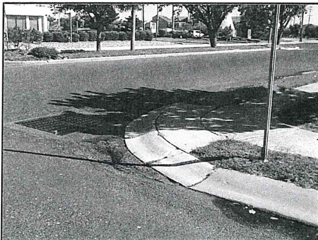
Curb ramp appear to be non-ADA compliant
