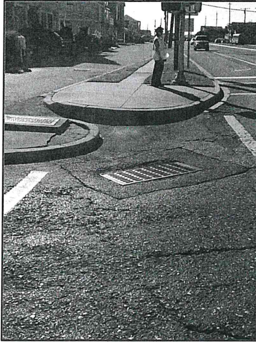
Curb ramp not ADA compliant
